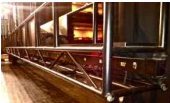
Electric Light Batten Structure
